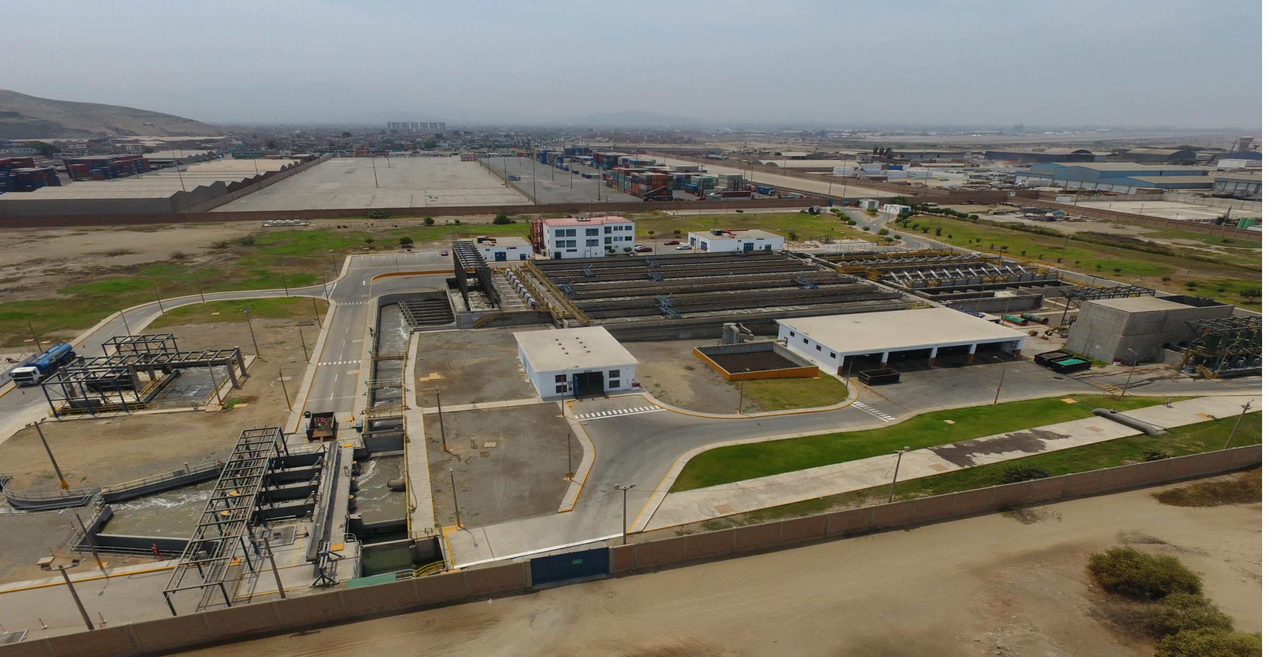
TABOADA WWTP - NORTHERN LIMA
