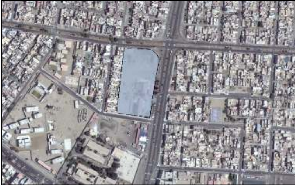
Picture 02: Location of the future Specialized Hospital of the Ancash Healthcare Network Source: Feasibility Study
