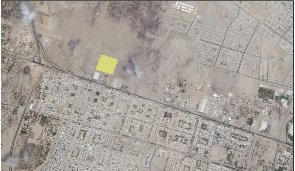
Picture 02: Location of the future Specialized Hospital of the Piura Healthcare Network
